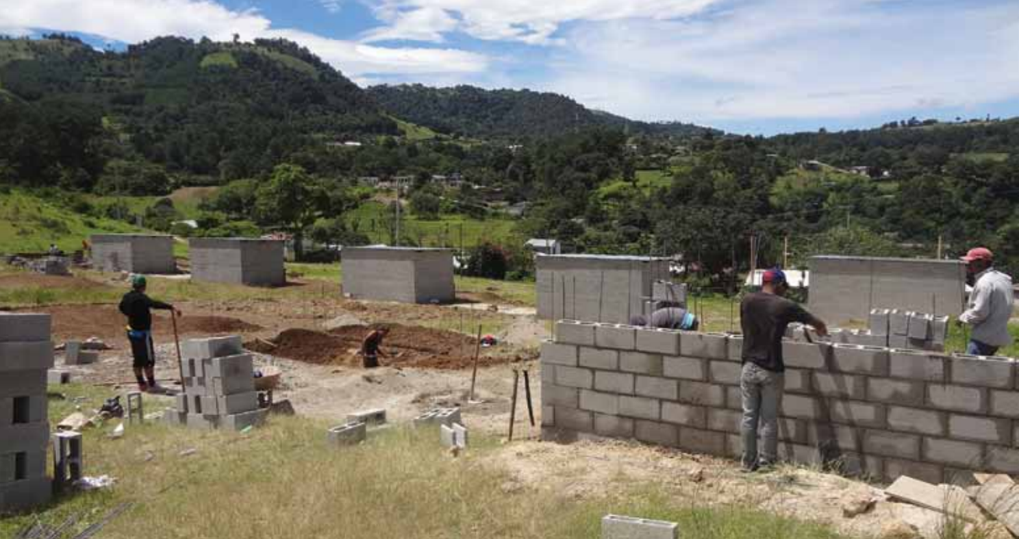
Houses in construction in Chutinamit
