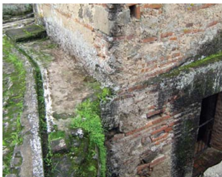
Water supply channel above the nuns' cells, part of a complicated hydraulic system
